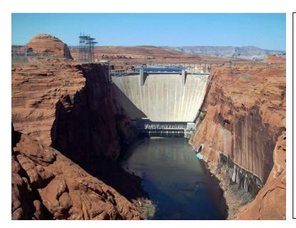
At 710-feet tall, this concrete archgravity dam near Page, Arizona, fills a canyon-heavy region on the upper Colorado River with water. Under construction from 1956 to 1966, the dam forms Lake Powell behind it, the second-largest man-made reservoir in the U.S.
