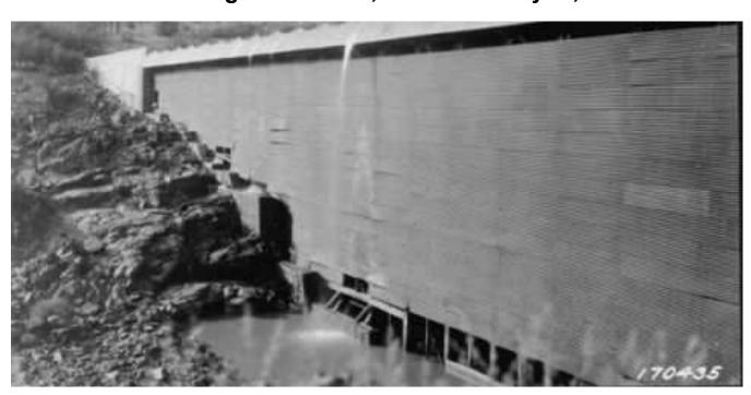
Almost everything about the Ashfork-Bainbridge Steel Dam is different than a typical dam in the West. Not only is it one of only two major dams in the nation using steel—the first of the two—this 1898-completed structure had no hydroelectricity generation purpose.
