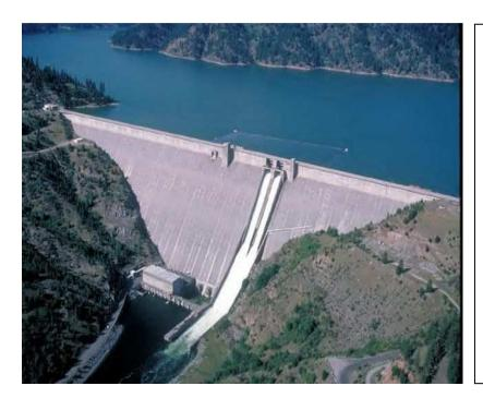
It took roughly seven years to build what would become the third tallest dam in the nation and the tallest straight-axis (not curved) concrete gravity dam in the Western Hemisphere. Dworshak Dam sits a few miles outside of Orofino, Idaho, blocking up the Clearwater River and creating the Dworshak Reservoice since 1973.
