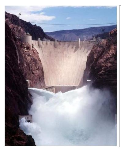
The superlatives fly when it comes to the Hoover Dam. Built between 1931 and 1935, the Art Deco-detailed dam was easily the most expensive engineering project in the country at the time and became the tallest dam in the country at 726 feet tall. Still the second-tallest dam overall and the tallest concrete dam, it required 91.8 billion cubic feet of concrete to create the arch-gravity dam with a 600ft-wide base, weighing 6.6 million tons in total.
