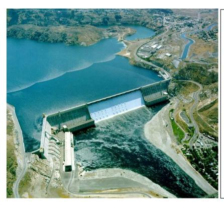
The Grand Coulee Dam may not be the tallest at 550 feet, but the seriousness of this 1942-built dam outside of Spokane, Washington, comes from its sheer size. With over 12 million cubic yards of concrete, the Ground Coulee Dam spans the Columbia River for nearly a full mile, backing up Franklin D. Roosevelt Lake reservoir nearly to Canada.
