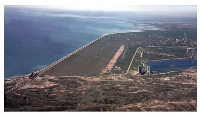
Forget the concrete and don't worry about the height. At just 250 feet tall, the impressiveness of the Missouri River's highest dam comes in its breadth. At over 21,000 feet in length and with a base width of 3,500 feet, Fort Peck is the largest hydraulically filled dam in the world.
